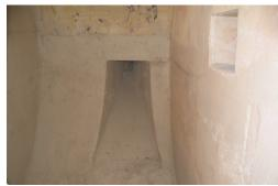
A tower melter lined with Capiral 85XS showing minimal deterioration after 12 months service.
